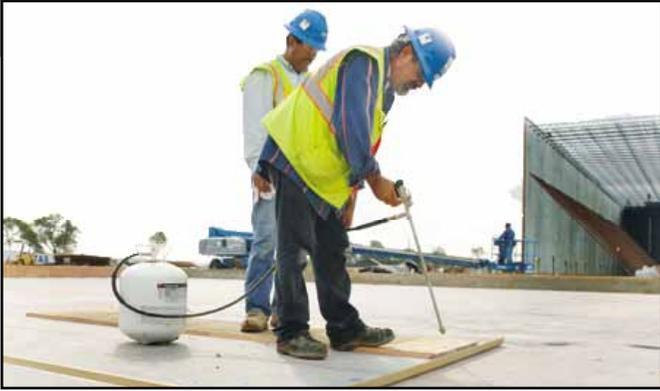
Hot melts are an alternative to some solvent-based adhesives for quick bonding.
